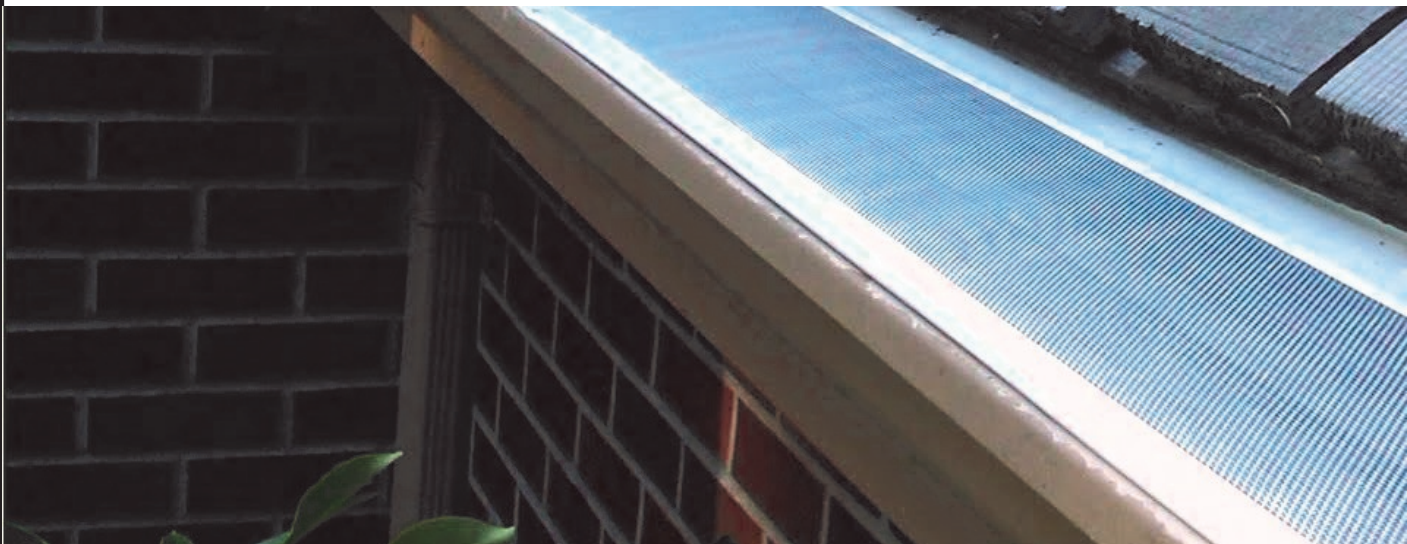
These aluminum and stainless steel gutter covers look appealing and are functional
